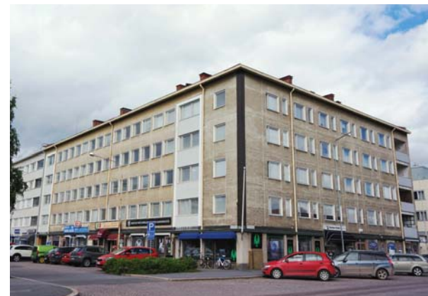
④⑧ AS OY ASEMAN SILTA
